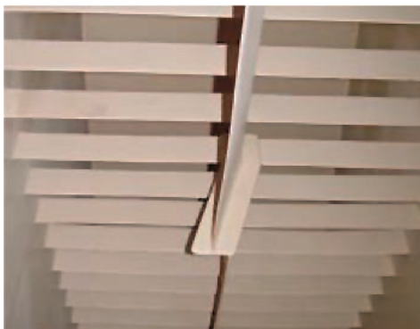
Clean gas duct deflecting plates
