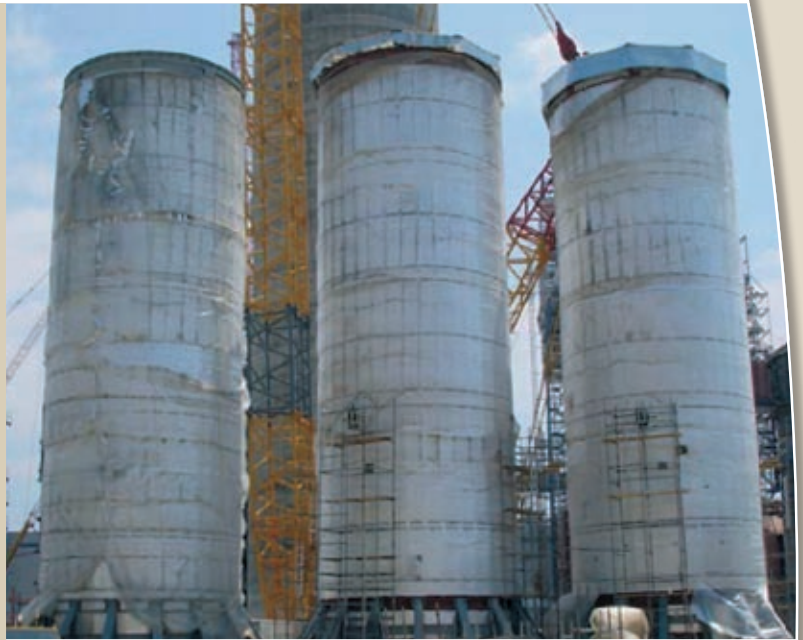
Prefabricated chimney stacks
